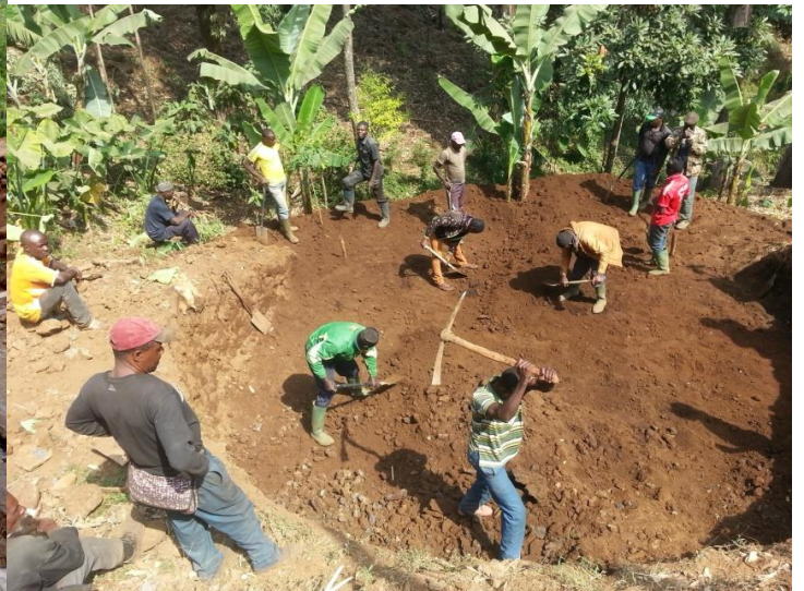
Storage tank site excavation in progress
