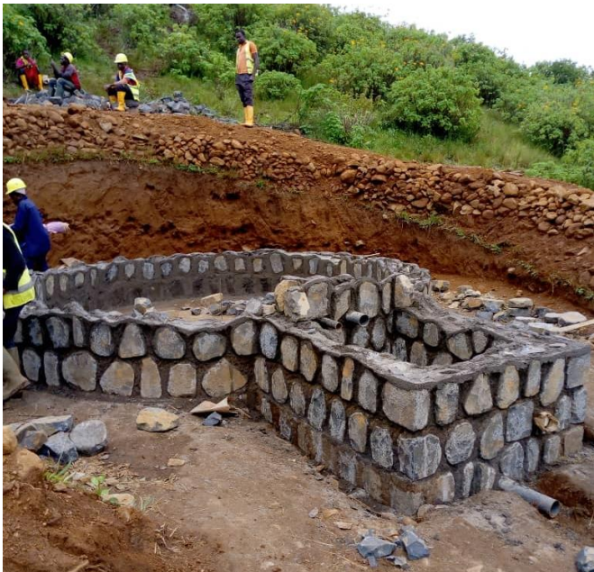
Storage tank under construction
