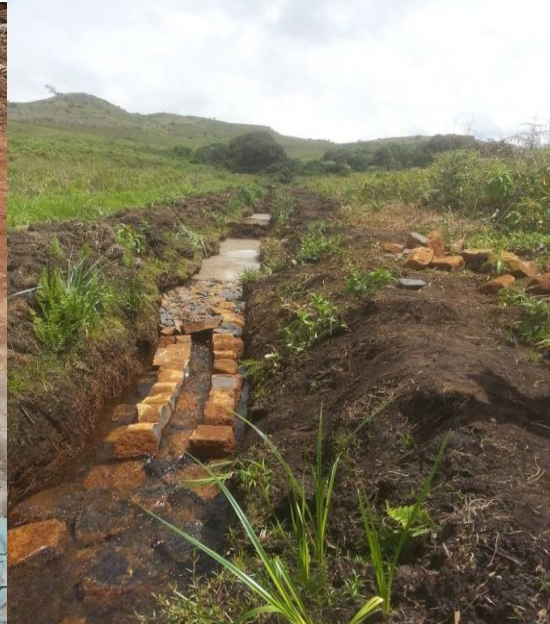
1.2Km Long Catchment Channel in progress
