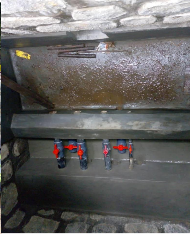
External and internal view of the catchment chamber with control valves just before completion
