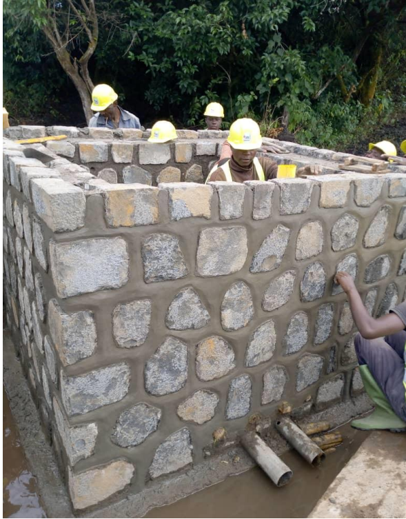
External and internal view of the catchment chamber with control valves just before completion
