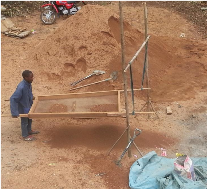
Grading of Sand, Storage tank site
